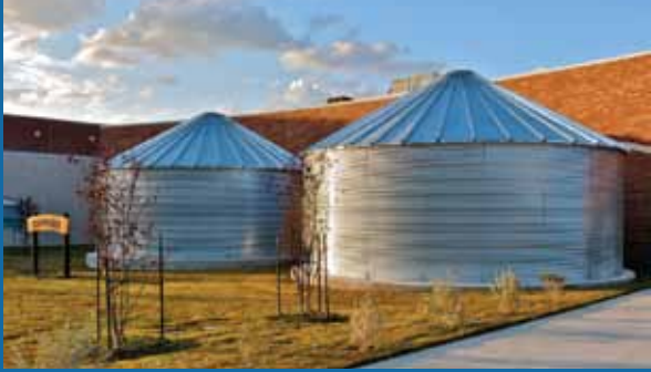
Carpenter Hill Elementary School, Buda, TX. 106,000 gallons of rainwater storage; photo by HarveyJack, wh 2 O.
