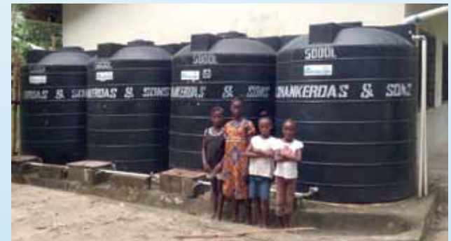
School, Makali, Sierra Leone. 20,000-liter rainwater storage for 90-inch annual rainfall. www.RainBank.info ; submitted by Ken Blair.
