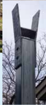
Austin, TX. Elegant fence is also an aqueduct, carrying rainwater overhead to cistern. www.loop-d.net , submitted by Christy Seals.
