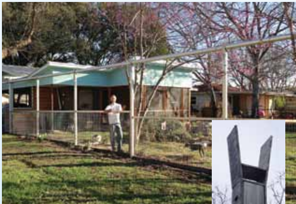
Austin, TX. Elegant fence is also an aqueduct, carrying rainwater overhead to cistern. www.loop-d.net , submitted by Christy Seals.
